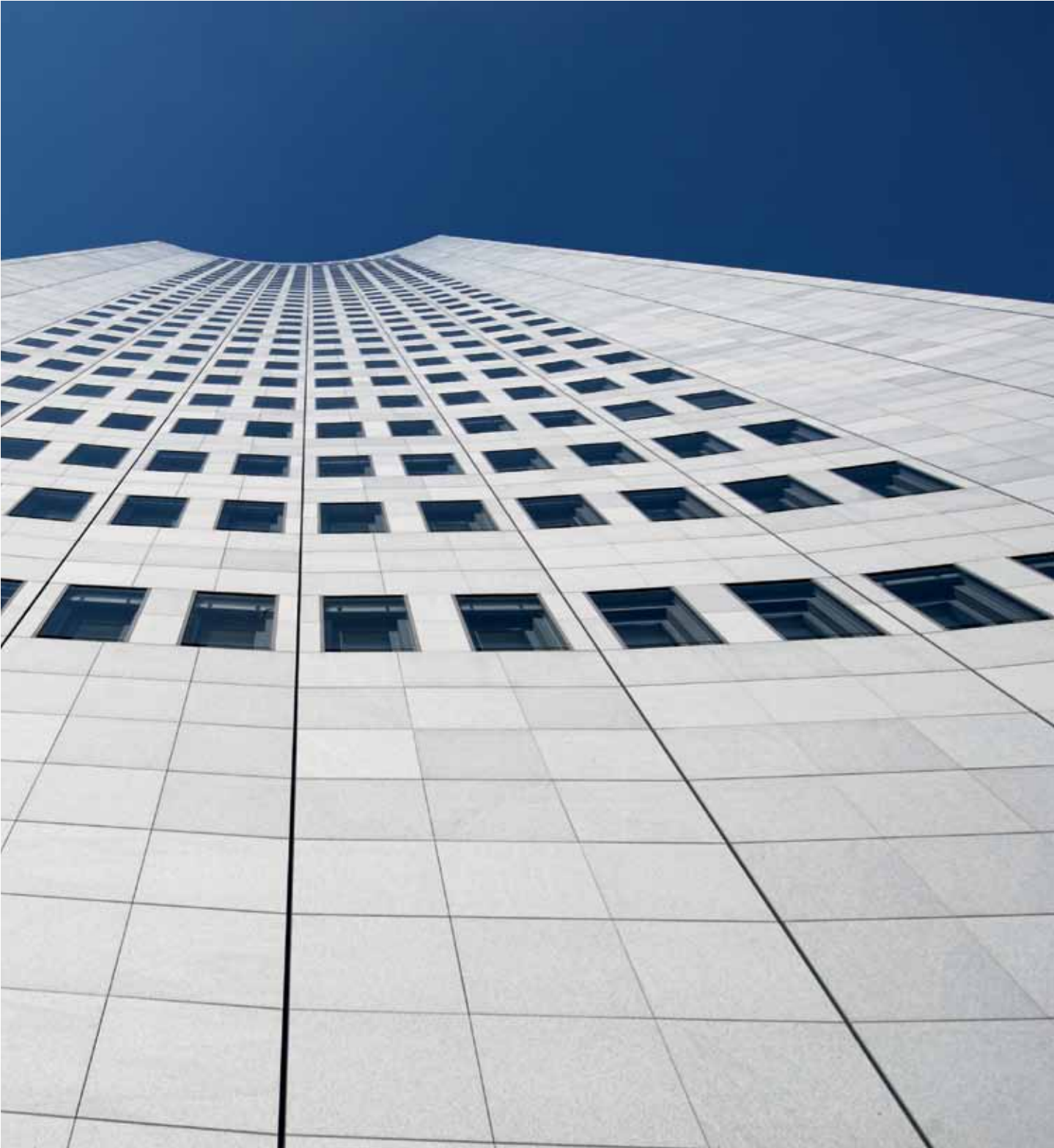
EEX corporate headquarters at Augustusplatz in Leipzig
